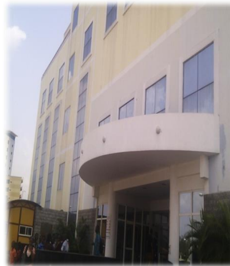
Figure 2: Exterior wall of the building with window openings Source: Author 2023
